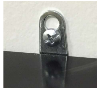
Top mounting shown in photo above with the seismic clip secured to the wall.
